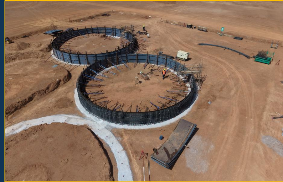
(R) Ring Beam Foundations
