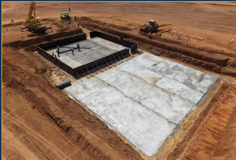
(R) Mill area raft foundation
