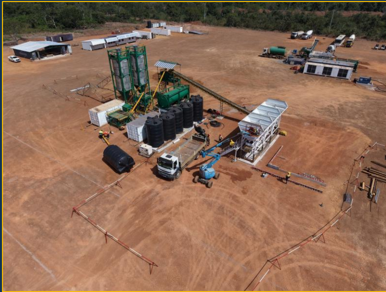
(L) Concrete batch plant commissioned
