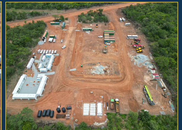
Contractor Laydown & construction Offices
