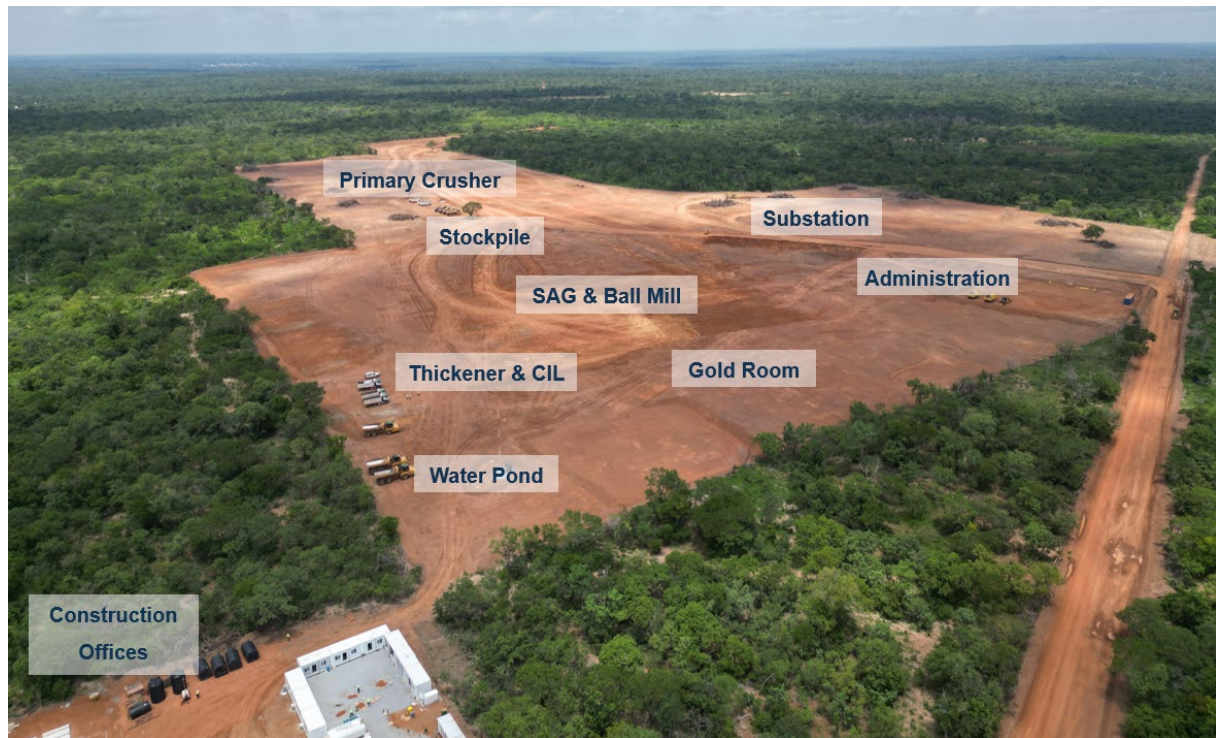
Figure 2: Site of Processing Plant
