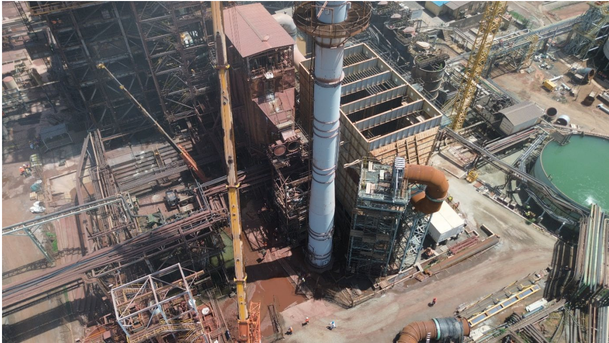
Figure 8: New Electrostatic Precipitator being tied in
