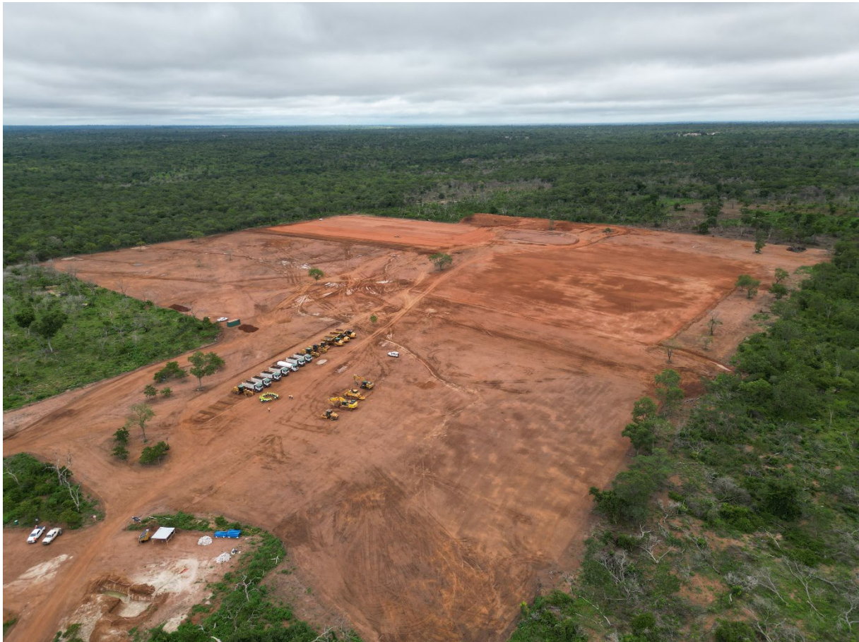
Figure 4: Construction Camp and Mine Village area
