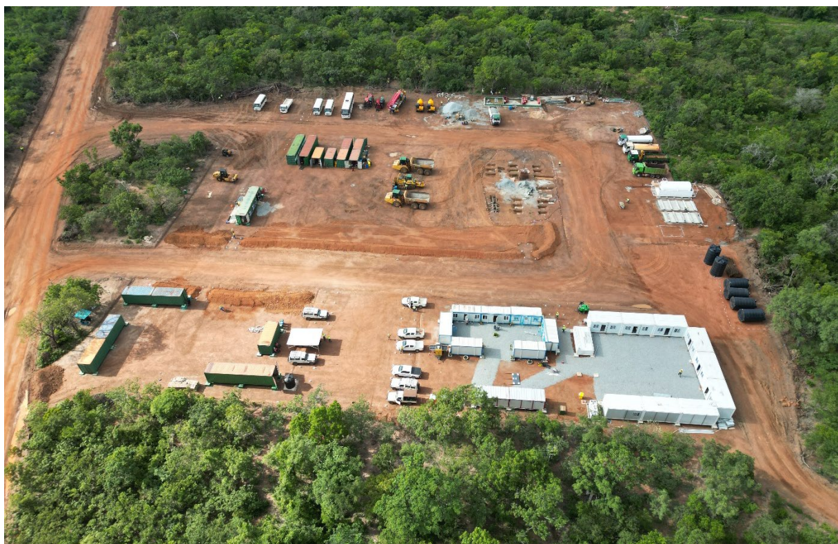
Figure 3: Contractor Laydown and Resolute Construction Offices
