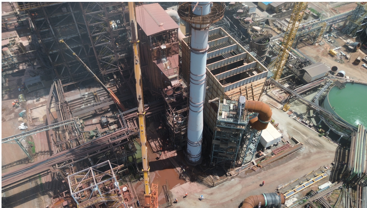
Figure 8: New Electrostatic Precipitator being tied in
