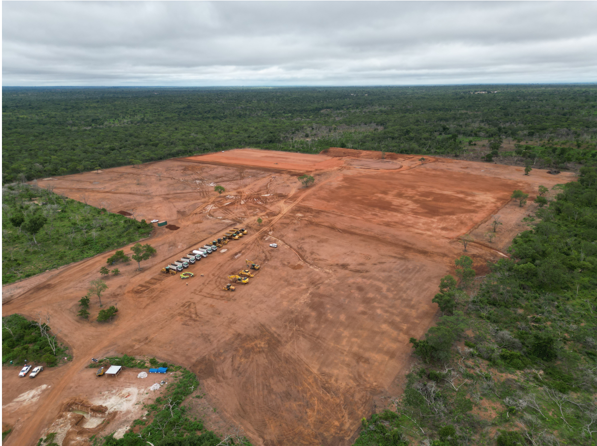
Figure 4: Construction Camp and Mine Village area
