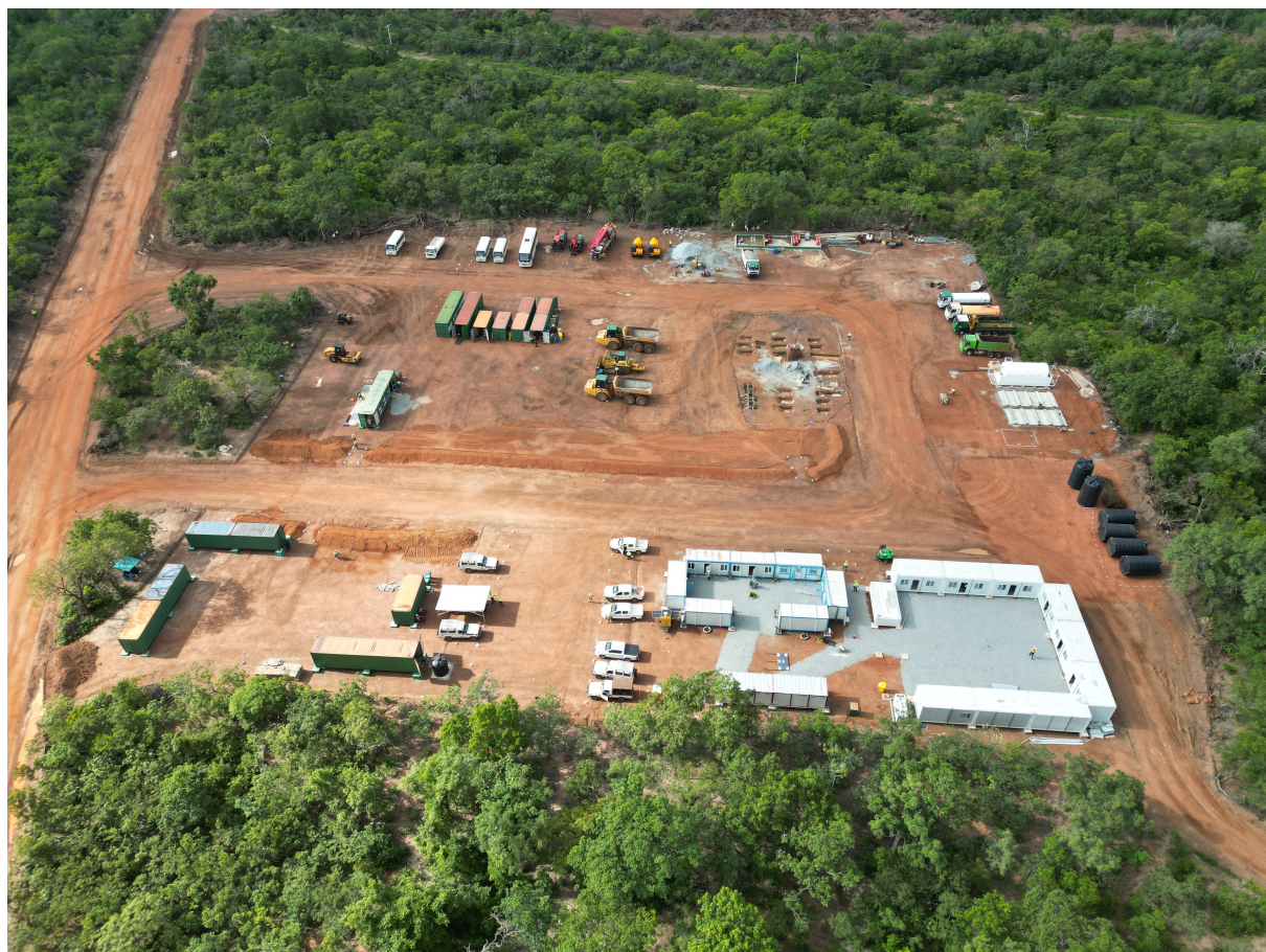
Figure 3: Contractor Laydown and Resolute Construction Offices
