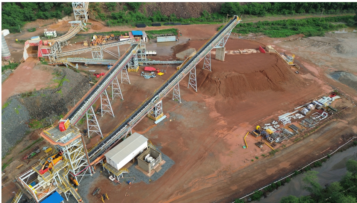
Figure 9: Secondary Crusher Circuit to be commissioned in Q3 2026
