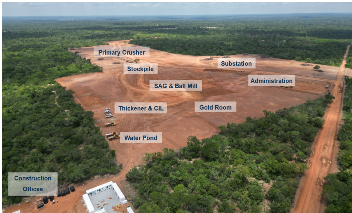
Figure 2: Site of Processing Plant
