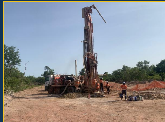
Borehole drilling in progress at 96 metres depth
