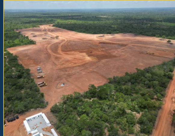
Process Plant Site Cleared
