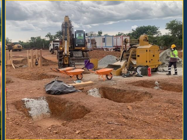
Blinding poured for workshop area
