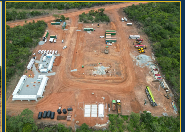
Contractor Laydown & construction Offices
