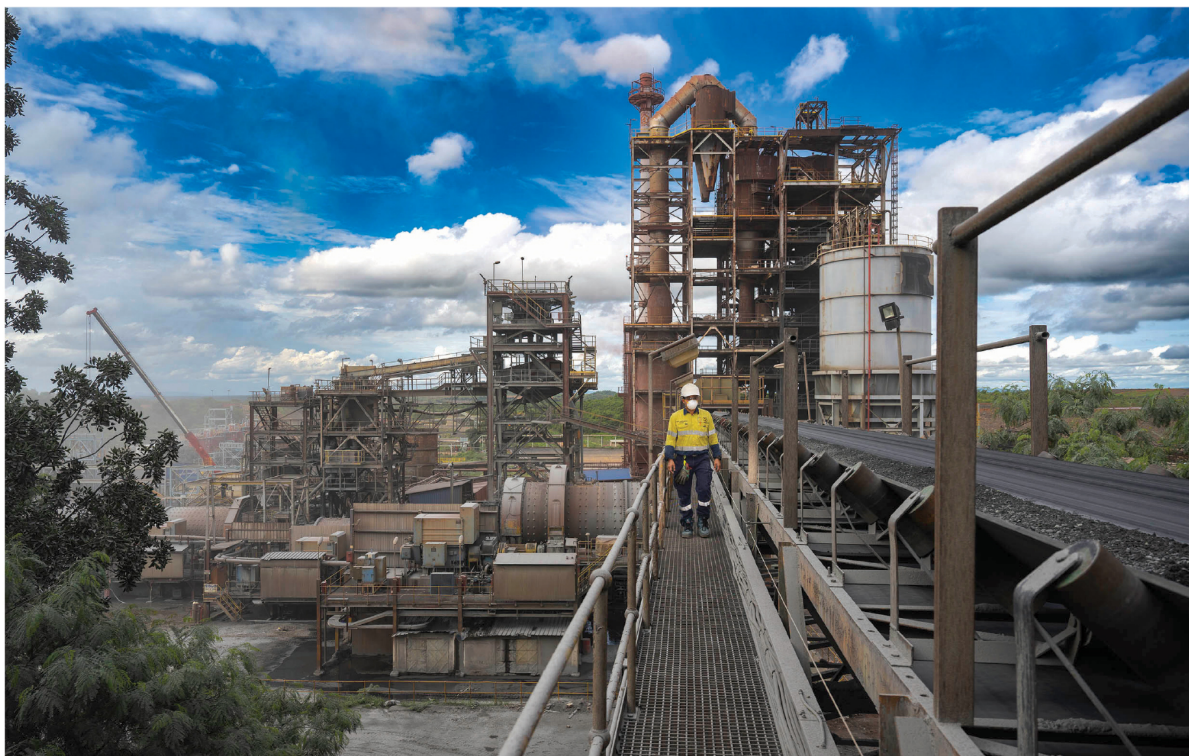
↑ The Syama processing plant. A project to increase sulphide processing capacity at Syama from 2.4 Mtpa to 4.0 Mtpa is nearly complete
