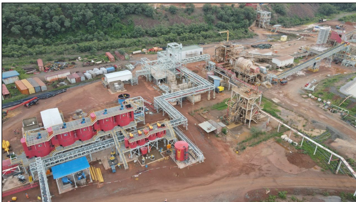
Figure 5: Ball mill and flotation areas
