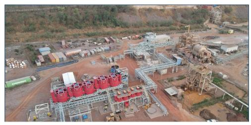
Ball mill and flotation areas under construction. The flotation circuit is now 86% complete, while the ball mill areas is 35% complete
