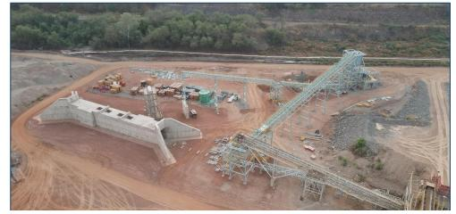
Secondary crusher and sulphide stockpile feed conveyor areas are 50% and 30% complete respectively
