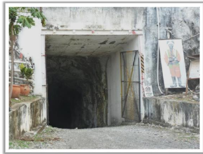
Figure 15.2 Existing portal and decline access located in the east wall of the Bibiani Main Pit
