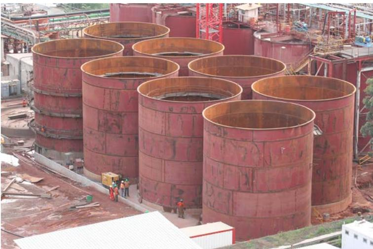
Figure 2. Oxide CIL tank erection October 2013
